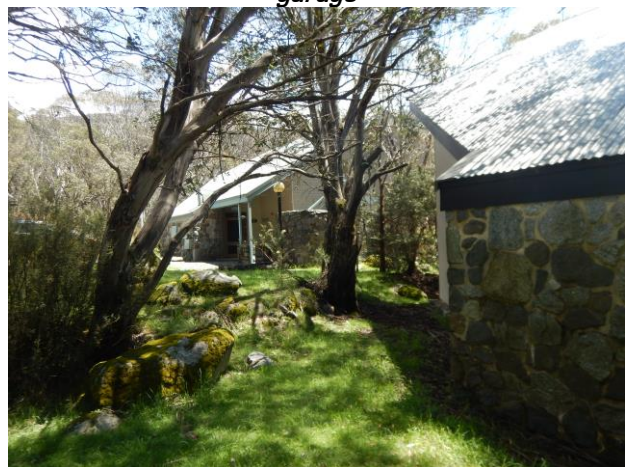
Figure 6: Photo of location for the proposed double garage – looking west
