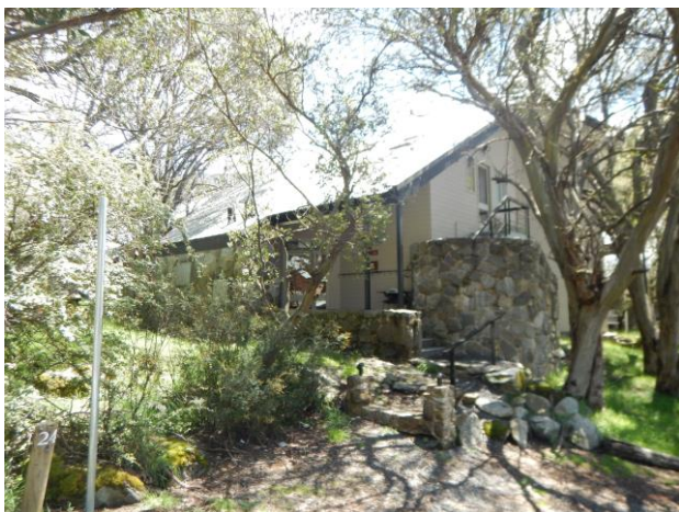
Figure 5: Photo of the existing entry to the chalet
